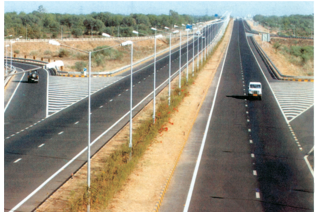
Fig.7.2: Ahmedabad- Vadodara Expressway
